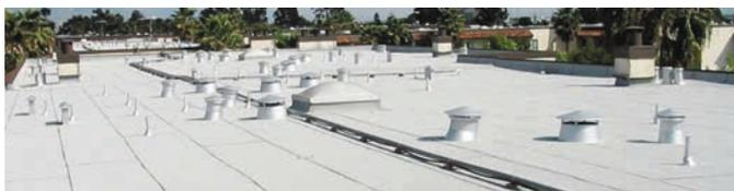
APP modified bitumen membranes are self-adhering when heated using a roofing torch. SBS modified bitumen membranes can be formulated for torch application, but are more commonly applied using hot asphalt or cold SBS modified bitumen adhesive. The result is a BUR system with significantly enhanced performance capabilities. Continuing improvements in technology have also resulted in self-adhering SBS roof membranes.
